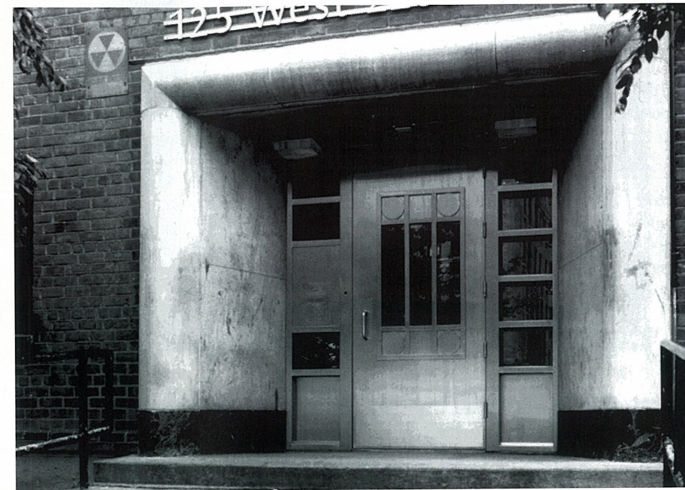
This heavy-gauge stainless steel door at New York's Marble Hill Houses was installed to ensure a long, trouble-free service life.
